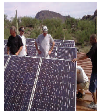
Solar Panel Installation training in Tucson, AZ.
